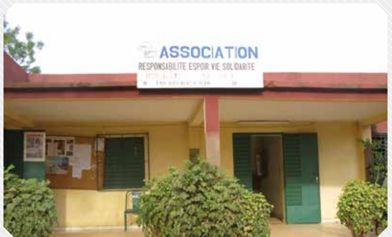
REVS+ head office, Bobo Dioulasso
